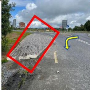
Area Traversable due to Grasscrete and signs in sockets.
